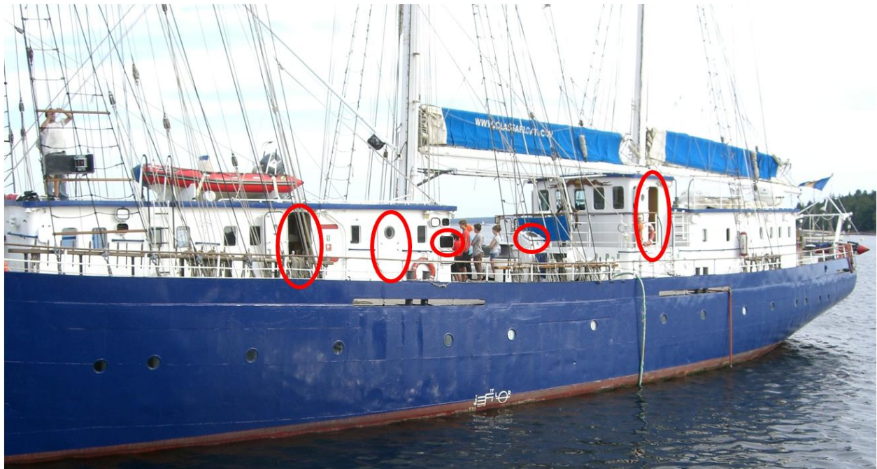
Photo 3. Some critical port side openings
