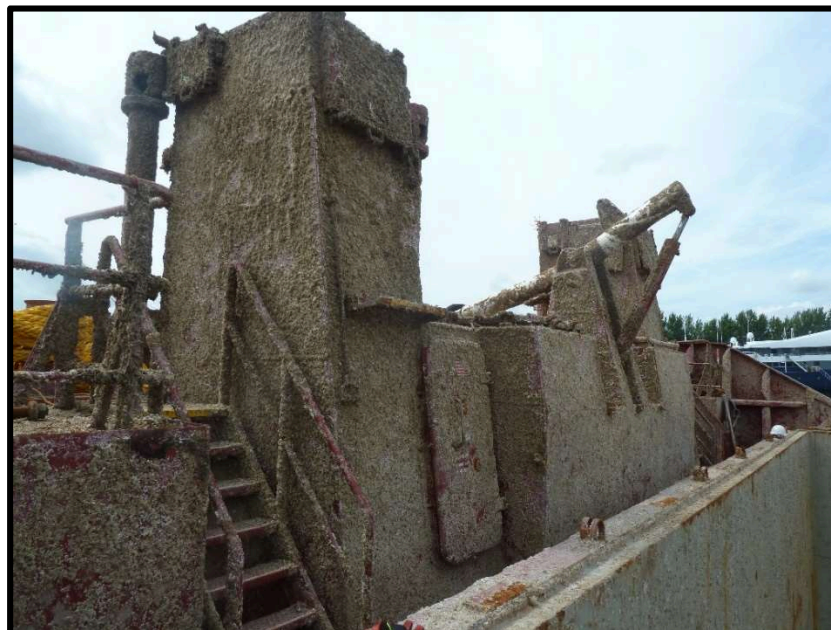
Fig 12: Cargo Hold Ventilators
