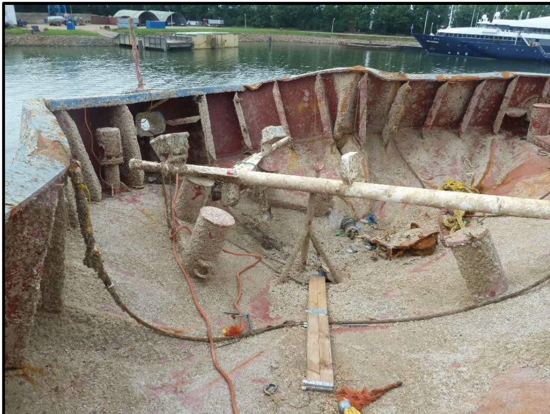
Fig 37 Damage to Focsle
