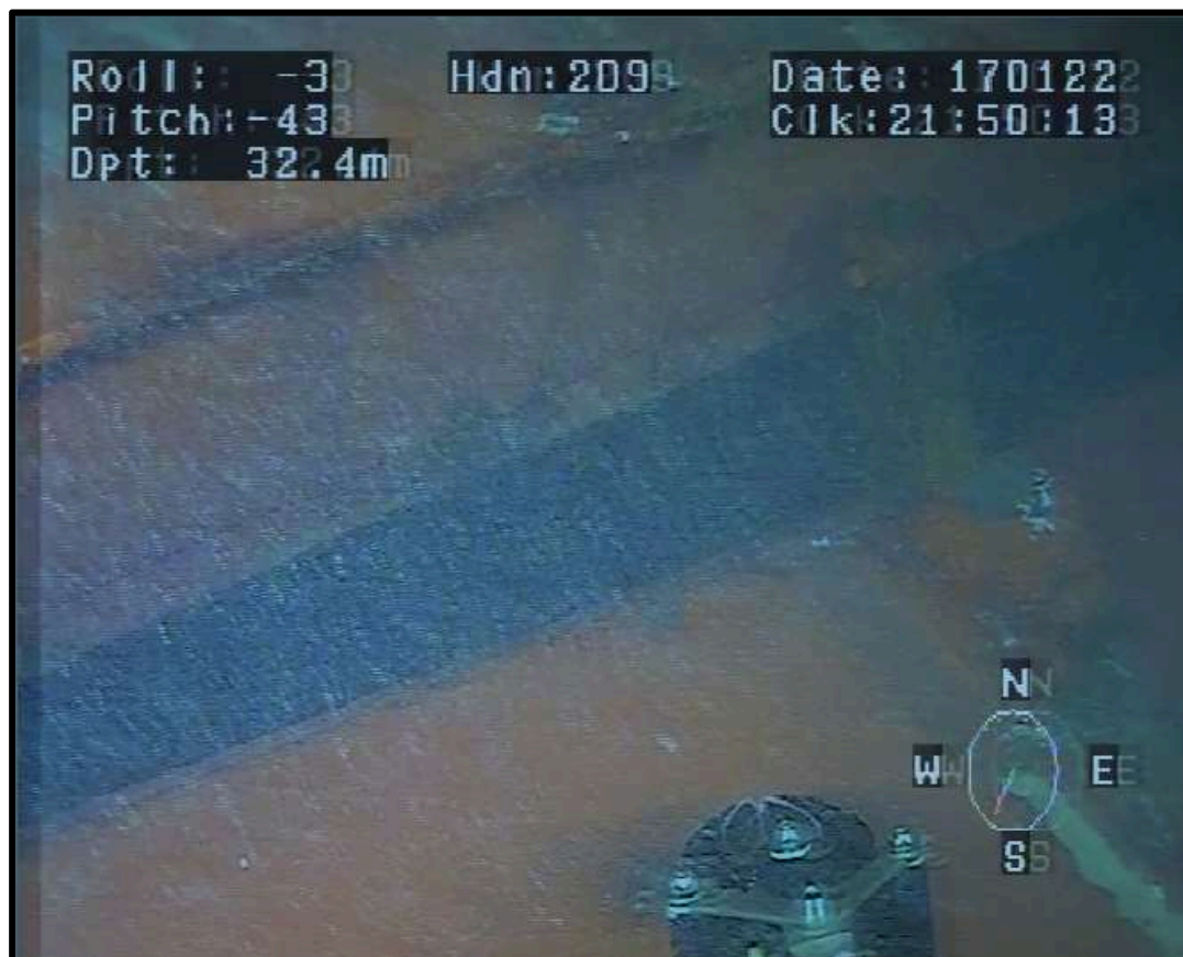
Fig 33 Distorted No. 3 hatch cover
