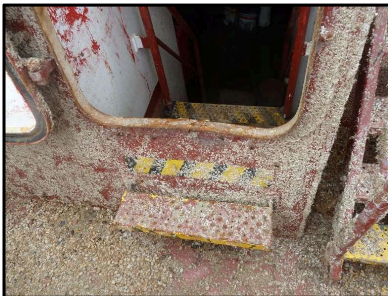
Fig 29 Focsle Door – distorted bottom of frame
